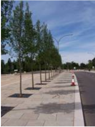
A45 Urban Boulevard – under construction
