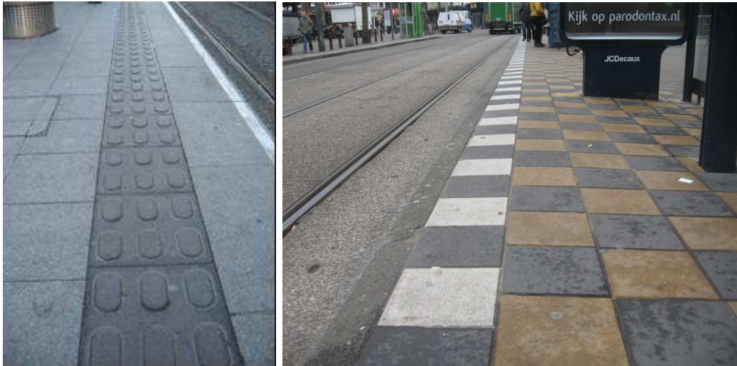
Plate 4.12 Best practise lozenge paving in Dublin (left) and good colour contrast at tram stop in Remandtplein, Amsterdam (right)
