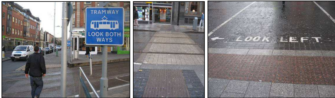
Plate 4.10: Signage and surface markings can improve the legibility of a crossing
