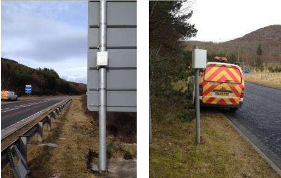
**Figure 4.1: Typical Bluetooth Sensor Installations**
